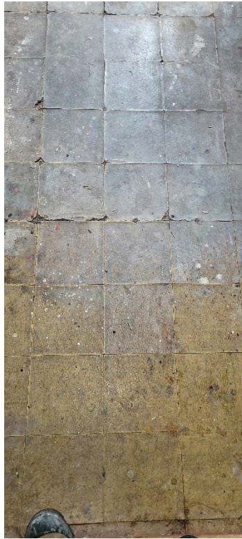
Photo 15: Floor of storage room – 9x9 tiles
