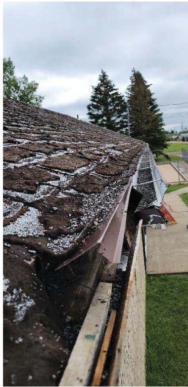
Photo 9: Roof edge and gutters Southside
