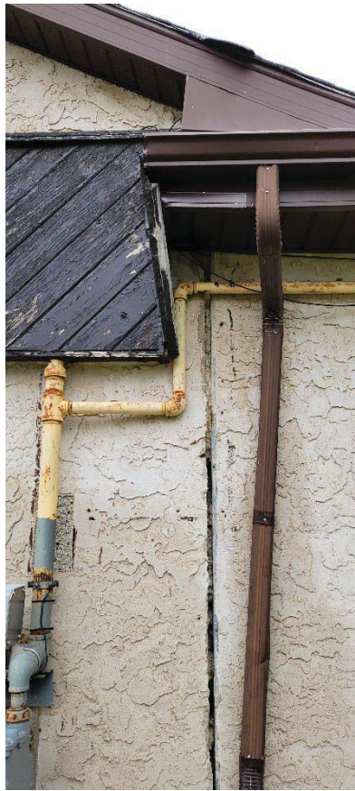
Photo 5: Building separation between North & South wings
