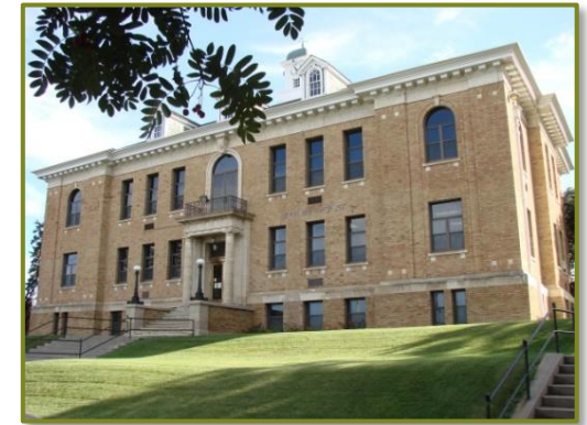
Prince Albert Court House photo courtesy of City of Prince Albert
